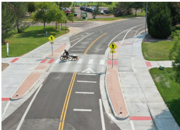
Raised crosswalk for trail crossing
