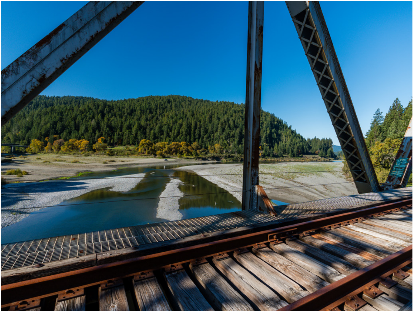
Dyerville Train Truss Bridge over Eel River near Founders Grove
