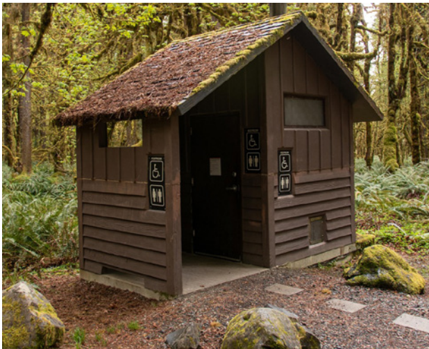
Backcountry Restroom - Vault toilet with structure (NPS)
