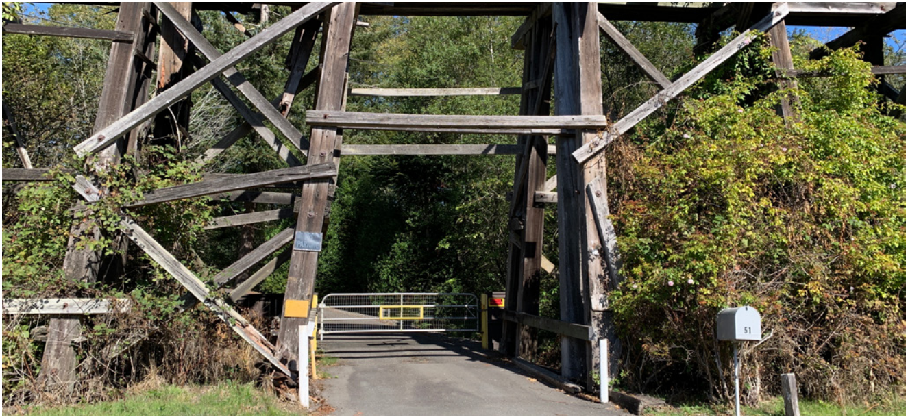
Existing private driveway
