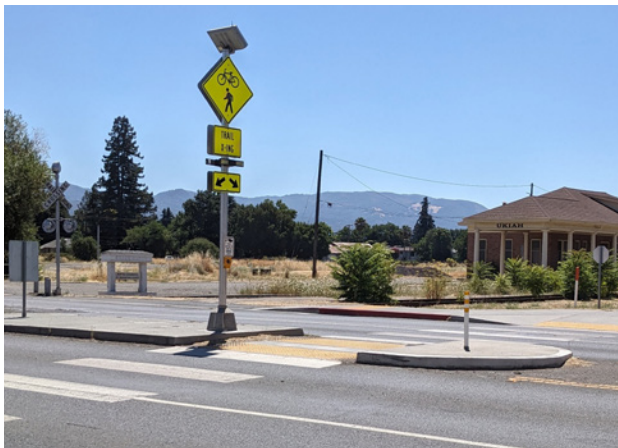
Existing pedestrian refuge island in Ukiah
