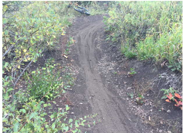
Natural Surface Crossings - drainage sheet flows across trail
