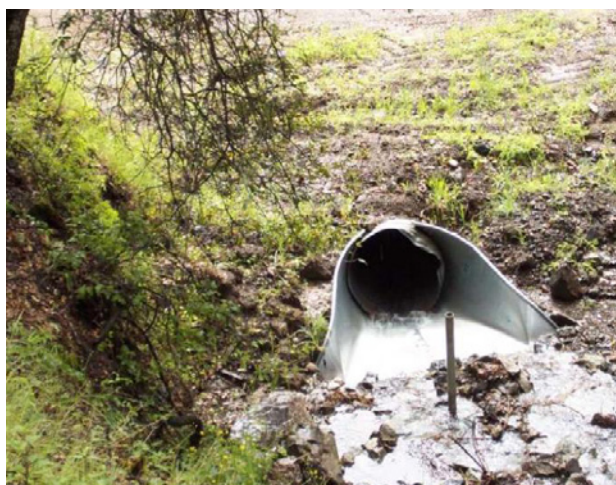
Flared culvert inlet
