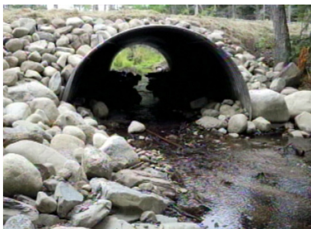
Arched Culvert with Stream Bottom
