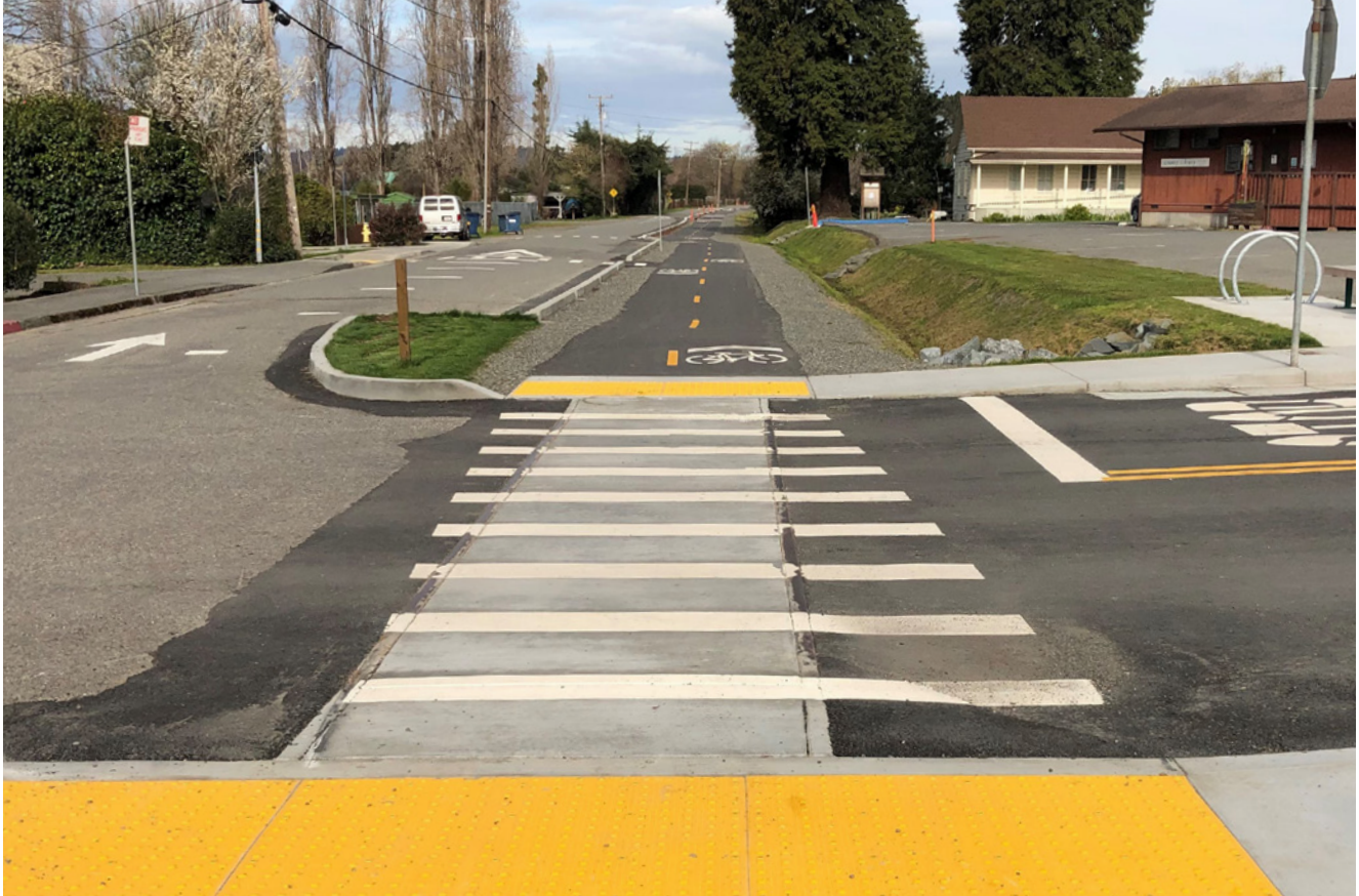
Existing trail crossing in Blue Lake
