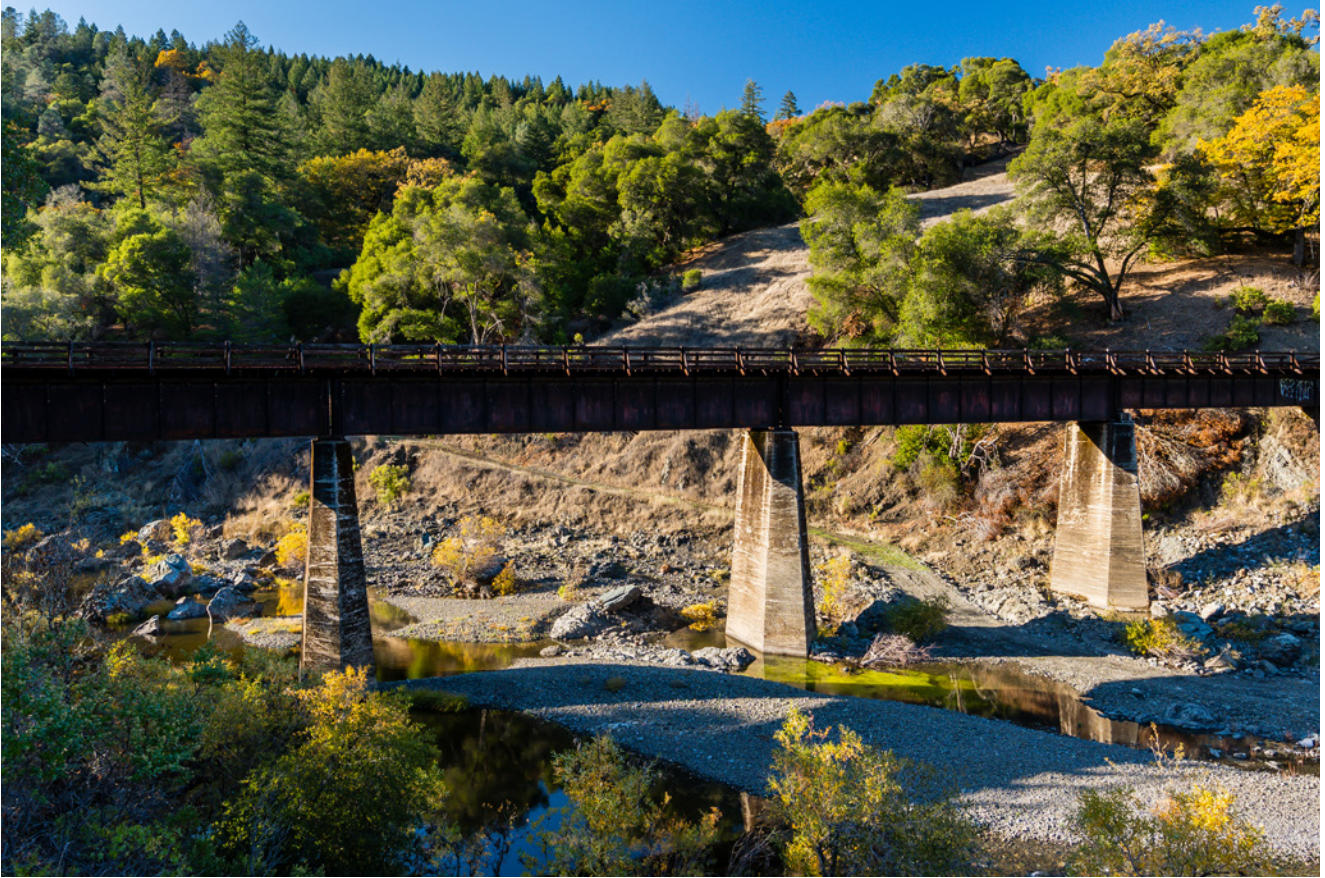
Former Northwestern Pacific Railroad Bridge over Outlet Creek
