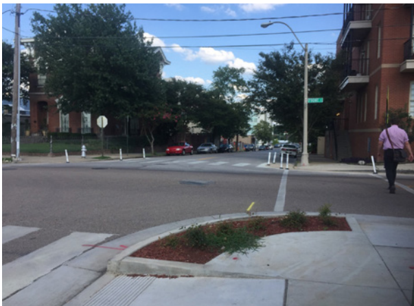
Tightened curb radius at pedestrian crossing
