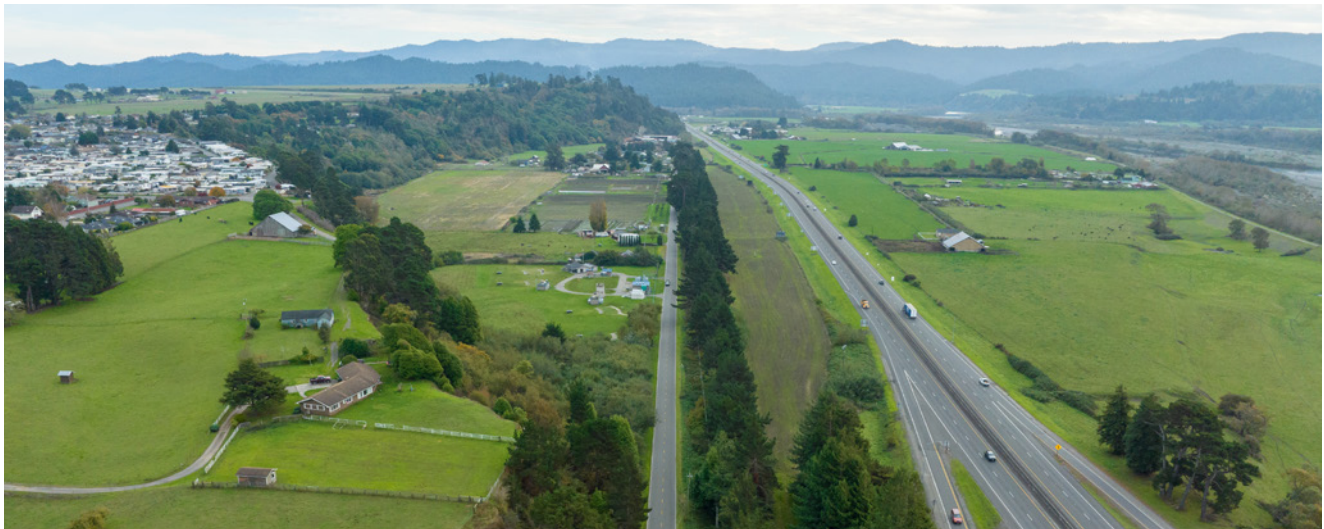
Overgrown GRT corridor south of Fortuna
