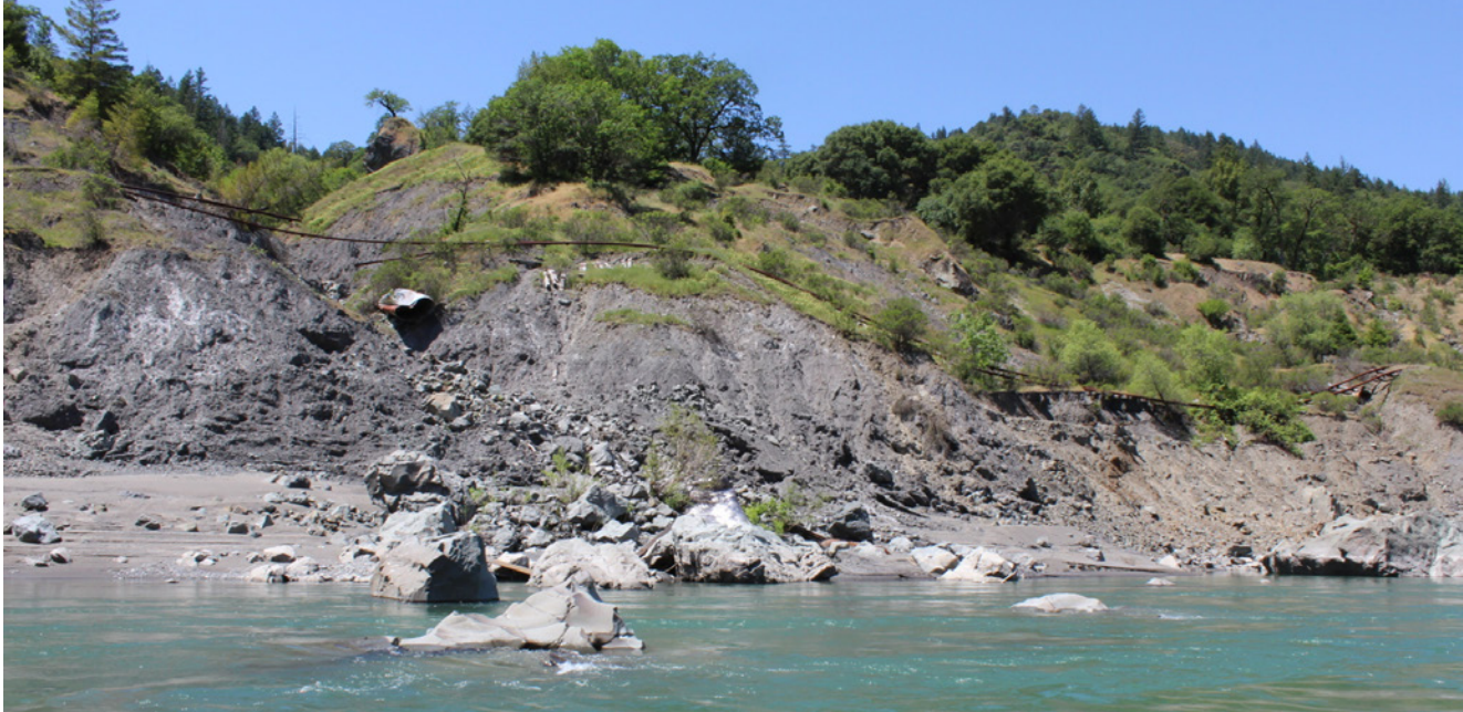
Washout of corridor with suspended track
