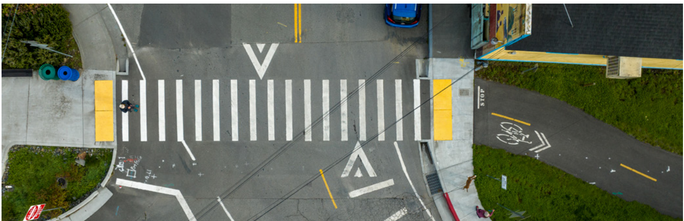
Existing trail crossing in Blue Lake
