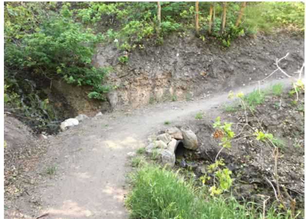
Small culvert at trail crossing
