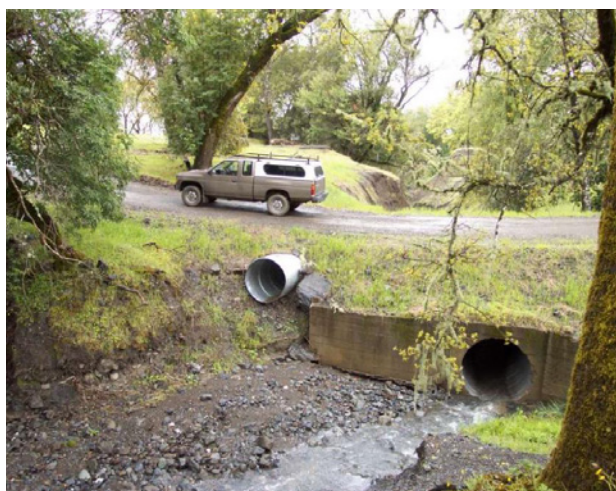
Emergency overflow culvert next to primary culvert
