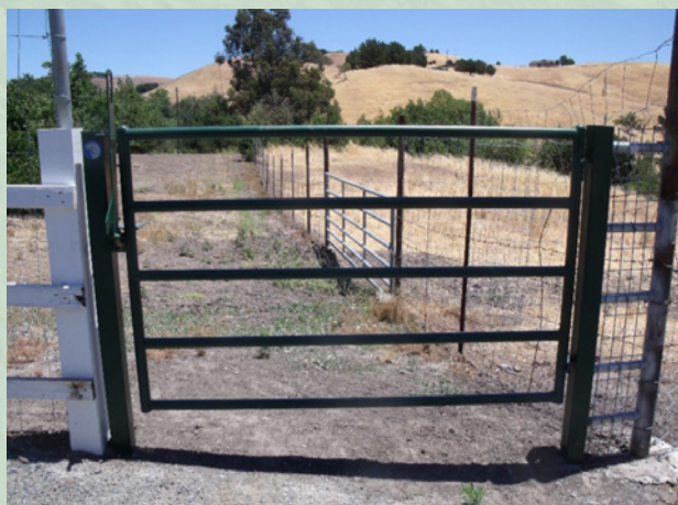
Self-closing pipe gate on EBRPD trail with livestock
