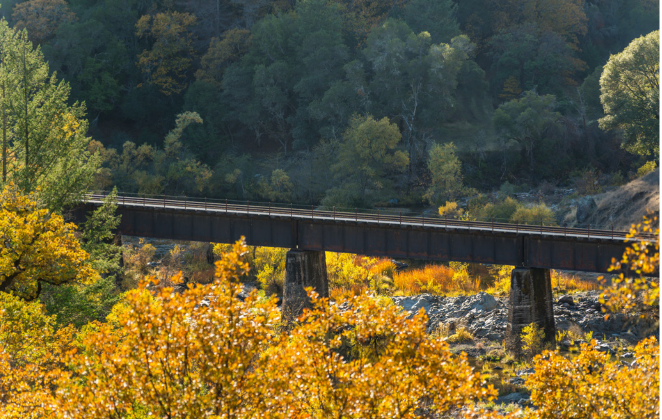
Existing bridge over Outlet Creek
