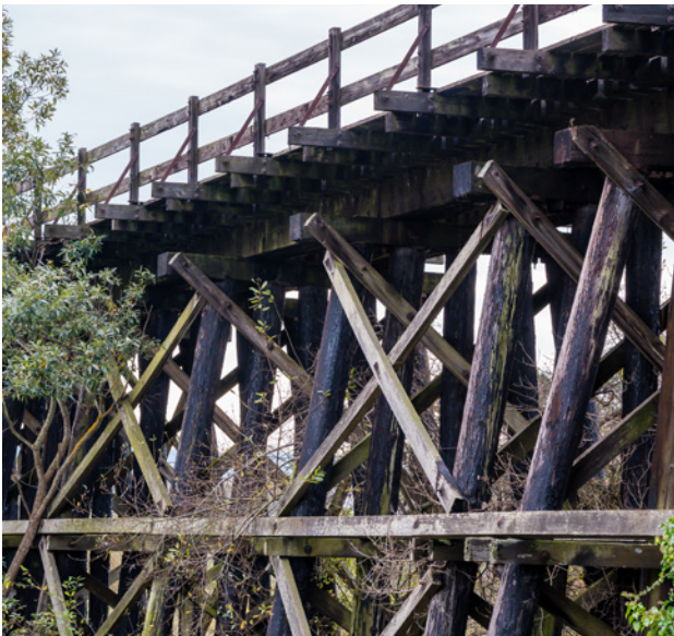
Existing trestle in Loleta
