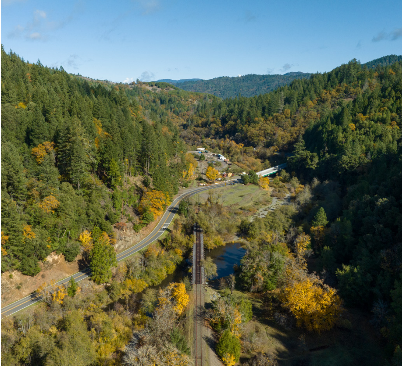
GRT corridor along Outlet Creek near Longvale
