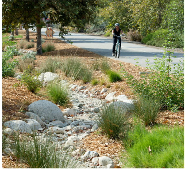
Bio-swale along a trail
