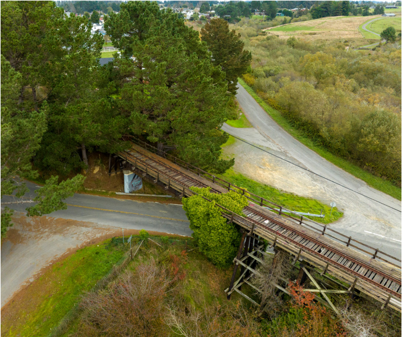
Railroad trestle near Loleta
